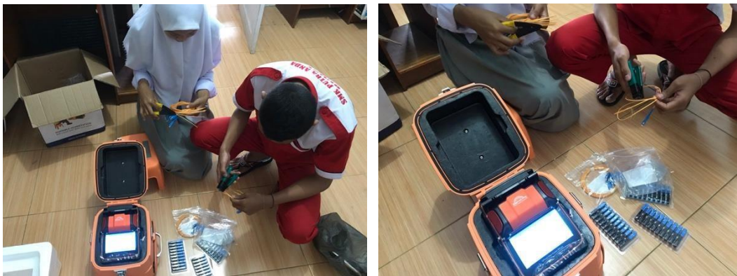
Gambar 3.2 Proses Pemasangan Fast Connector Fiber Optic
